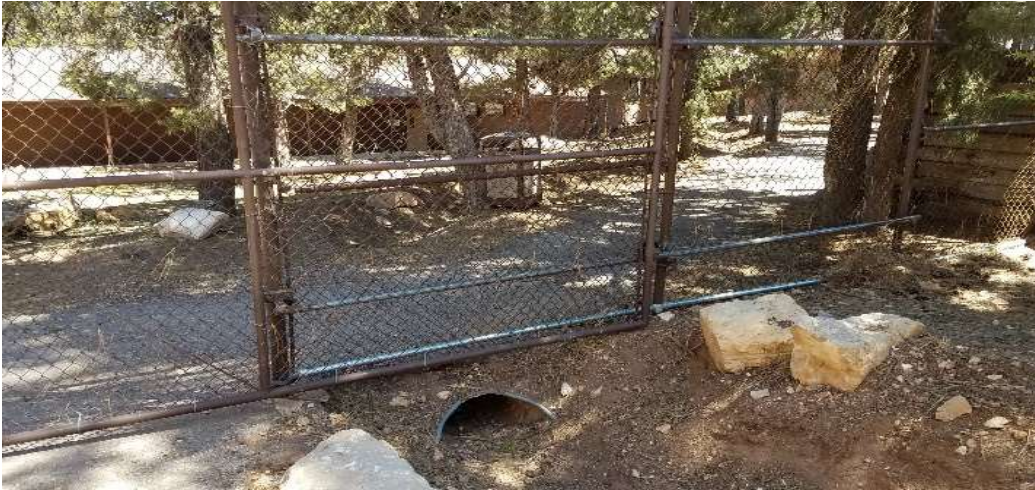
Figure 4: Example of culvert on site [3]
