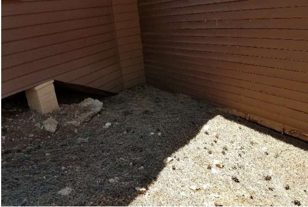
Figure 7: Example of surface flow causing erosion [3]
